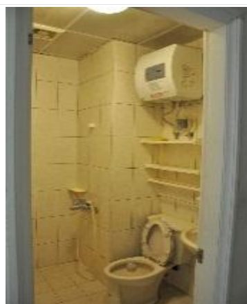
Bathroom (in each room)
